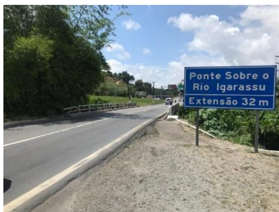
Fig. 1: Top view of the bridge
