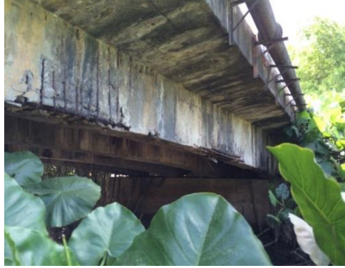
Fig. 7: Infiltrations, efflorescence and generalized staining on the lower surfaces of the deck
