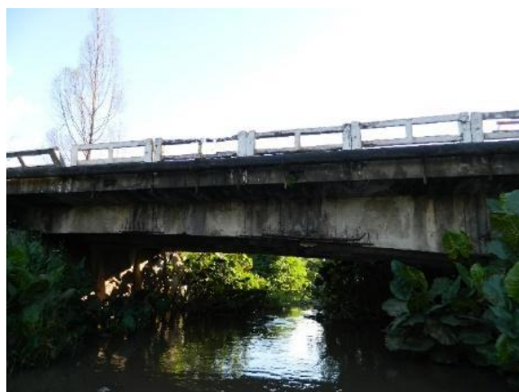
Fig. 2: Partial side view of the bridge
