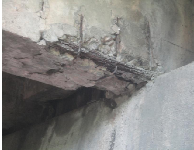
Fig. 5: Severe corrosion and destruction of shear reinforcement in regions of the external beams support
