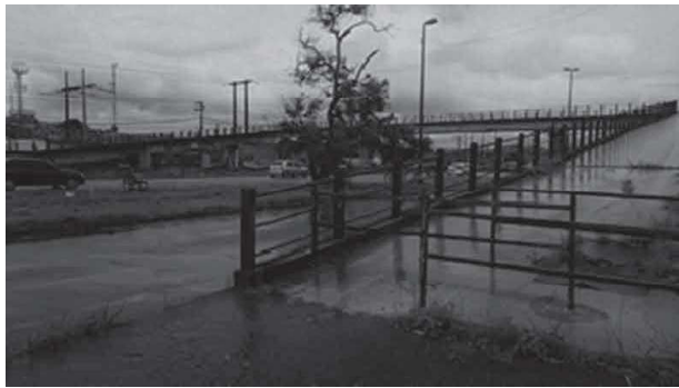
Figure 1. Longitudinal view of Curado walkway.
