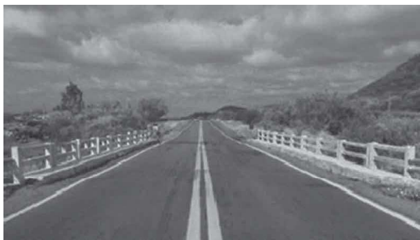
Figure 3. Top view of the bridge over the River Tanque.
